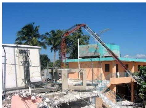
Figure 2a - damaged cell tower in PaP
