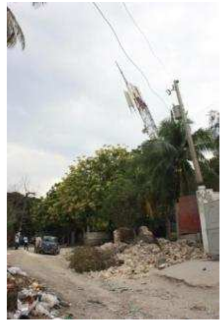
Figure 2b - Damaged cell tower in PaP
